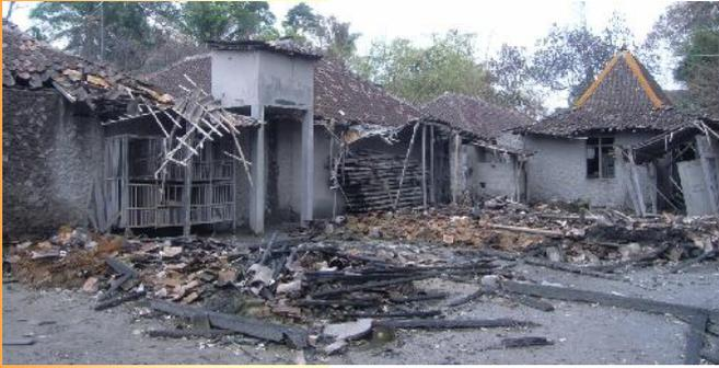
*Structural damage to buildings in Bronggang village, Argomulyo. Two timber frame buildings have suffered fires and collapses. The intact nature of tiles on the roofs, along with other evidences, suggests that this surge was associated with relatively low dynamic pressures.*
